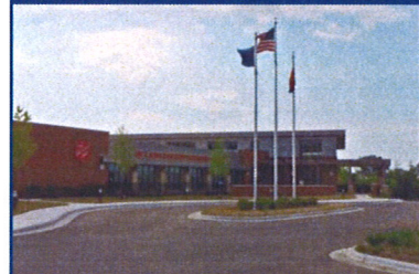
The Design of the Kroc Center Incorporated Innovative Retention Basins for Stormwater Conservation
